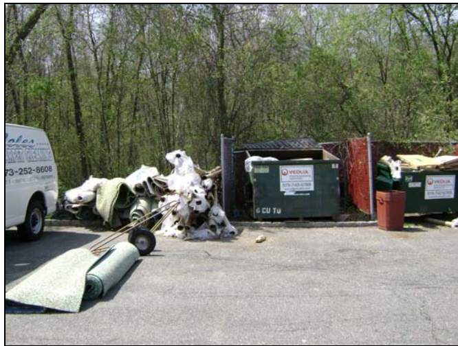
Figure 14: Dumpsters on construction site
